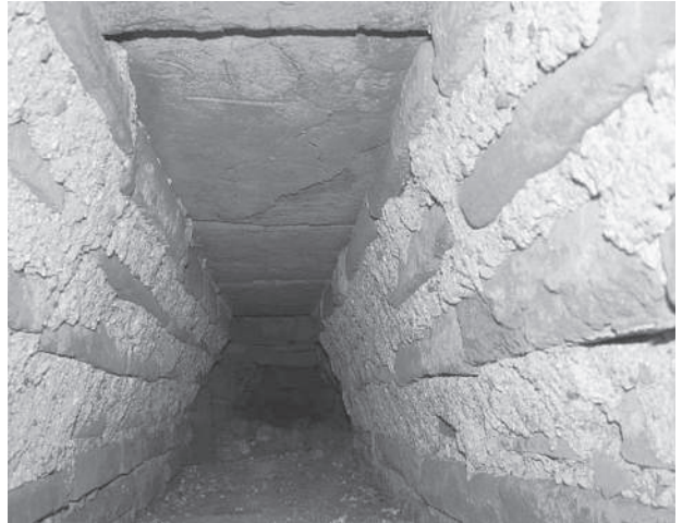
Res. 5 1 nolu sondajda ortaya çıkan hypokaust sistemi Fig. 5 Hypocaust system uncovered in sounding no. 1
